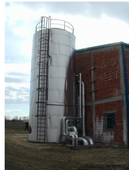
Akumulator toplote 100m 3
